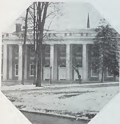
GRAHAM MEMORIAL BUILDING STUDENT UNION
